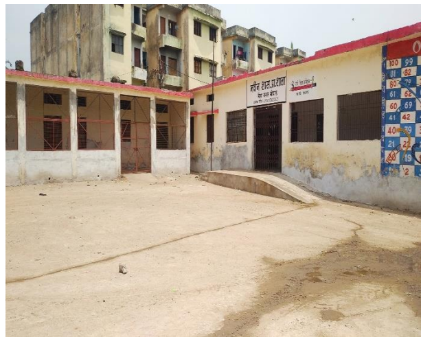
Meera Nagar Primary School after construction.
